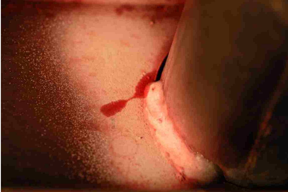
Figure 66. Specimen #2, crack at east weld of the S9-T1 intersection
