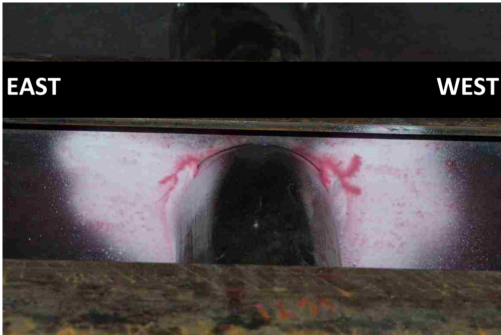
Figure 64. Specimen #1, cracks at S7-T1 intersection, shown with dye penetrant
